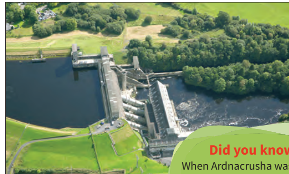
Fig. 16.02.12 The hydroelectric power plant at Ardnacrusha, on the River Shannon.
