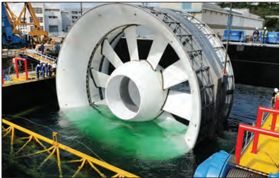
Fig. 16.02.06 Tidal turbine machine being installed.
